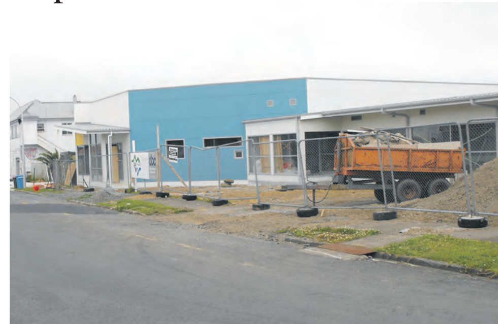
The construction site of the new health centre on Napier Street is now showing a bit of colour.
